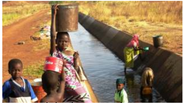
Irrigation water also serves domestic needs
