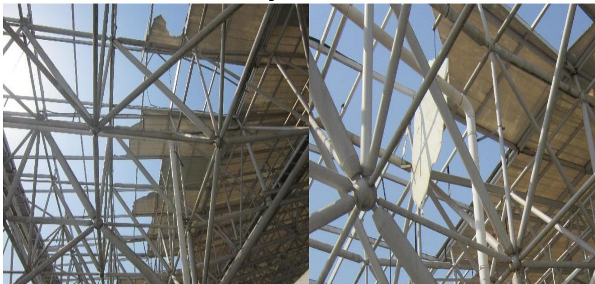
Picture 6: Portions of the roof at Essipon Stadium
